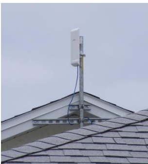
Figure 29 Typical WiMAX Installation
