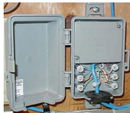
Figure 3 POTS/DSL Splitter
