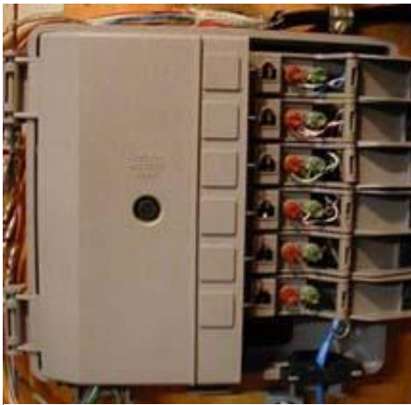
Figure 19 Network Interface Device
