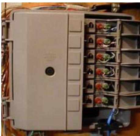
Figure 21 Network Interface Device
