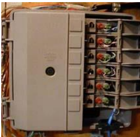
Figure 30 Typical Telco Demarc
