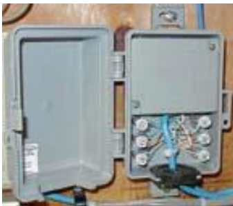
Figure 31 Whole House POTS/DSL Splitter
