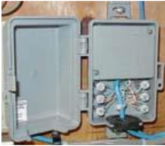
Figure 32 Whole House POTS/DSL Splitter
