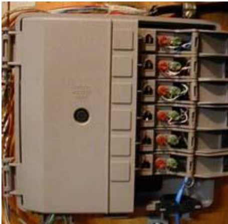
Figure 31 Typical Telco Demarc
