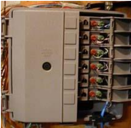
Figure 27 Typical Telco Demarc
