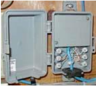
Figure 28 Whole House POTS/DSL Splitter
