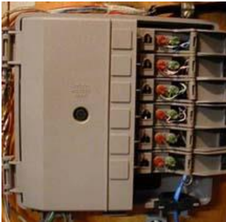
Figure 25 Typical Telco Demarc
