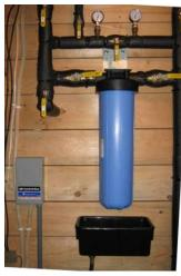
Pressure tank and sediment filter are located in the basement. Cold well water causes condensation on the pressure tank and filter housing. When I installed the system though I was being clever and decided to use the sediment filter as a poor man's dehumidifier.
